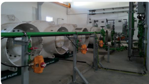
The plant has a modular design and each process stage is made up of a number of lines operating in parallel, a layout which facilitates maintenance.
