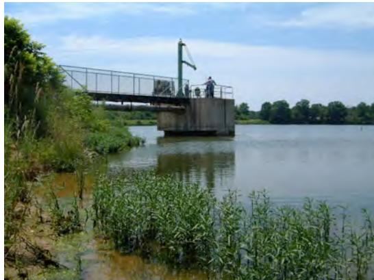
Shallow lake intake withdraws water at 12-foot depth close to shore
