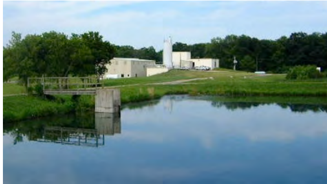
Greenville has a comprehensive water treatment plant sited on the shore of Governor Bond Lake
