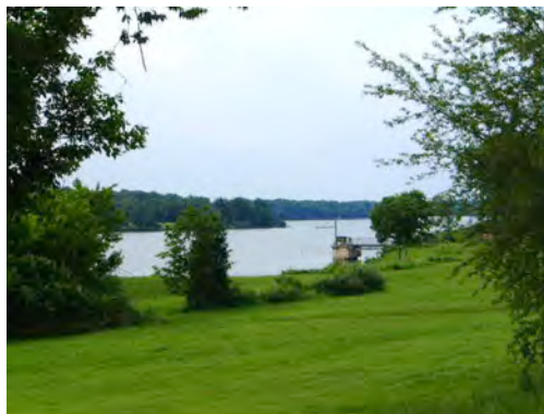
Governor Bond Lake showing near-shore water treatment plant intake structure
