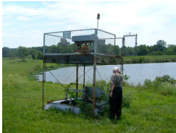
Destratifier removed from service for resuspending sediments
