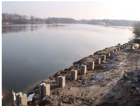
Construction of seawall to protect shoreline along Lake Bloomington
