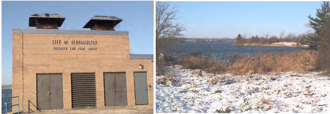
Pumping facilities at Evergreen Lake - High lake stage due to rain and snow, December, 2004
