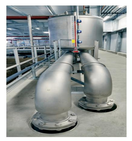
Variable-flow software lowers costs by automatically regulating flow into the dissolved air flotation tank through dual saturators Photos: CDM
